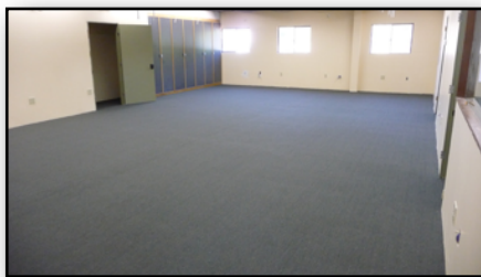
Meeting room after carpet installed.—photo by, Dave Illich,
